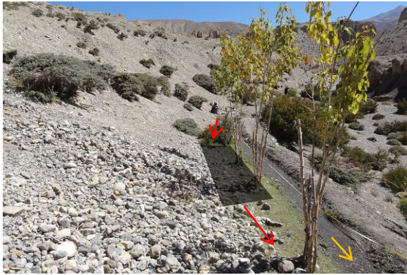
Figure 7.9: Position of the inspection chamber I2 ( x = 388 \text{ m} ; 29^{\circ}05'20.04''\text{N} / 84^{\circ}00'32.12''\text{E} ). Left: The pipeline (red arrows) and the chamber (black rectangle) are proposed to be shifted slightly inwards to be at a safe distance from the instable slope downhill. The open, earthen channel is highlighted by the orange arrow (photo: 27/09/2013, Daniel Bernet). Right: Bird's eye view of the inspection chamber's location. The red line indicates the pipeline and the yellow arrow points in Puyung Khola's flow direction (source: Google Earth Pro, accessed 30/01/2014).
