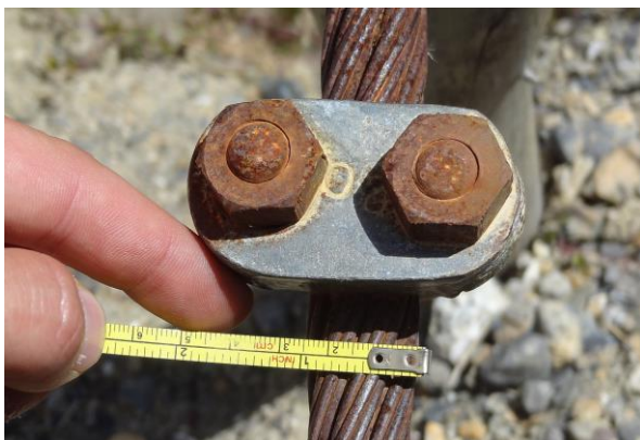
Figure 7.7: Proposed method to attach the pipeline to the steel rope. Left: To the anchor blocks of the crossing C1 and C3, a 25 mm steel rope is fixed. To attach the pipeline to the rope, 10 mm steel ropes and appropriate clamps, like the ones depicted in the photograph, are recommended (photo: 29/09/2013, Daniel Bernet). Right: cross-sectional sketch of the attachment method. First a small loop (orange arrow) at one end of the thin steel rope should be formed and fixed tightly with clamps. The rope should then be looped around the transversal steel rope and the pipeline. Following, the thin steel rope's loose end should be laced through the before created loop and tightened. The loose end should finally be looped back, fixed with clamps and the surplus rope should be cut.
