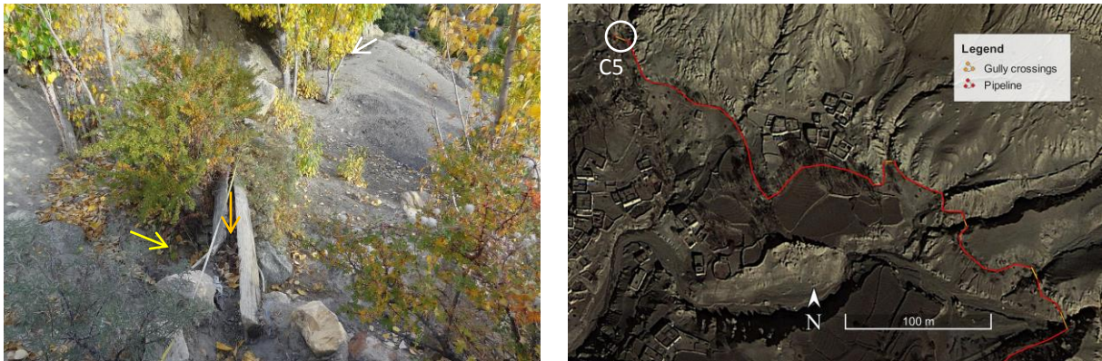
Figure 7.19: Position of the gully crossing C5 ( x = 2127 - 2134 m; 29^{\circ}05'47.41''N / 83^{\circ}59'58.05''E ). Left: The open channel (white arrow) is connected to a log with a carved-in slot (orange arrow), spanning over the small gully, indicated by the yellow arrow (photo: 27/09/2013, Daniel Bernet). Right: Marked location of the gully crossing (source: Google Earth Pro, accessed 31/01/2014).
