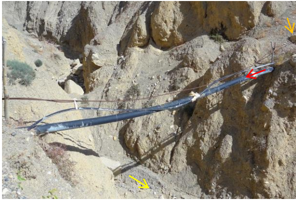
Figure 7.17: Position of the gully crossing C3 ( x = 1769 - 1781 m; 29^{\circ}05'43.40''N / 84^{\circ}00'06.67''E ). Left: The pipeline (red arrow) is attached to a steel rope, held by two concrete anchors, one of which is visible (orange arrow). The flow direction within the gully is indicated by the yellow arrow (photo: 26/09/2013, Daniel Bernet). Right: Marked location of the gully crossing (source: Google Earth Pro, accessed 31/01/2014).
