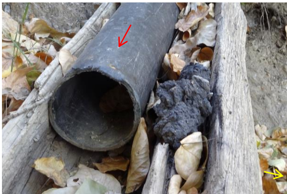
Figure 7.18: Position of the gully crossing C4 ( x = 1850 - 1854 m; 29^{\circ}05'44.70''N / 84^{\circ}00'04.75''E ). Left: The pipeline (red arrow) crossing the small gully (yellow arrow) rests on a wooden bar (photo: 27/09/2013, Daniel Bernet). Right: Marked location of the gully crossing (source: Google Earth Pro, accessed 31/01/2014).
