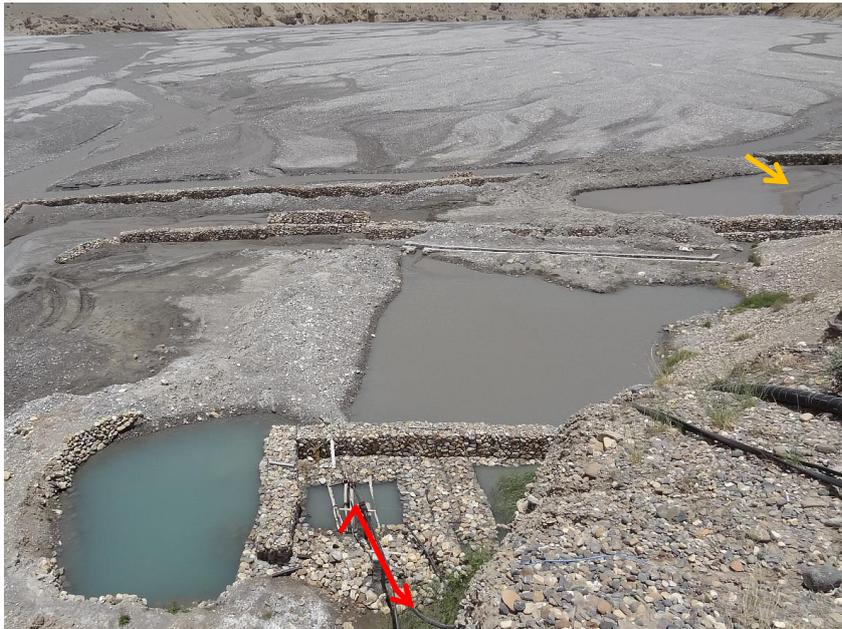
*Figure 5.3: A sequence of pools was installed to rid the water, abstracted from the Kali Gandaki (orange arrow), from suspended particles prior to pumping. Visibly, the water becomes much clearer before it is drawn in by the pump (red arrow). The water is lifted from the Kali Gandaki up to a vast plain near Tangbe, where an orchard is being cultivated. The pumps are connected to the power grid, which is currently not reaching much further up than Tangbe (photo: 21/06/2012, Daniel Bernet).*
