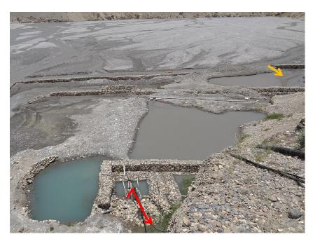
Figure 5.3: A sequence of pools was installed to rid the water, abstracted from the Kali Gandaki (orange arrow), from suspended particles prior to pumping. Visibly, the water becomes much clearer before it is drawn in by the pump (red arrow). The water is lifted from the Kali Gandaki up to a vast plain near Tangbe, where an orchard is being cultivated. The pumps are connected to the power grid, which is currently not reaching much further up than Tangbe (photo: 21/06/2012, Daniel Bernet).
