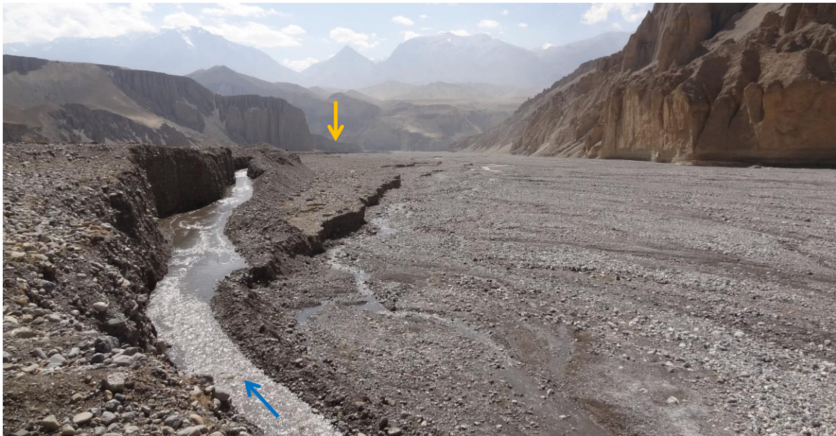
Figure 5.8: Existing water abstraction which is supplying the newly built orchard with water. The flow direction is indicated with the blue arrow. Due to high flow of the Dhey Chang Khola at the end of June, the intake was damaged and put out of operation. According to the local people, the intake will be reactivated in February next year. Thangchung, located roughly 2 km further downstream, is highlighted with an orange arrow (photo: 13/05/2012, Daniel Bernet).
