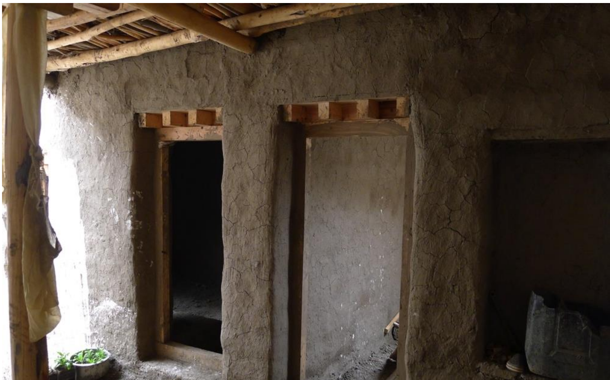
Figure 3.9: Inside view of a house in Dheye with earthen walls, wooden poles and wooden slab (photo: 05/07/2012, Daniel Pittet).
