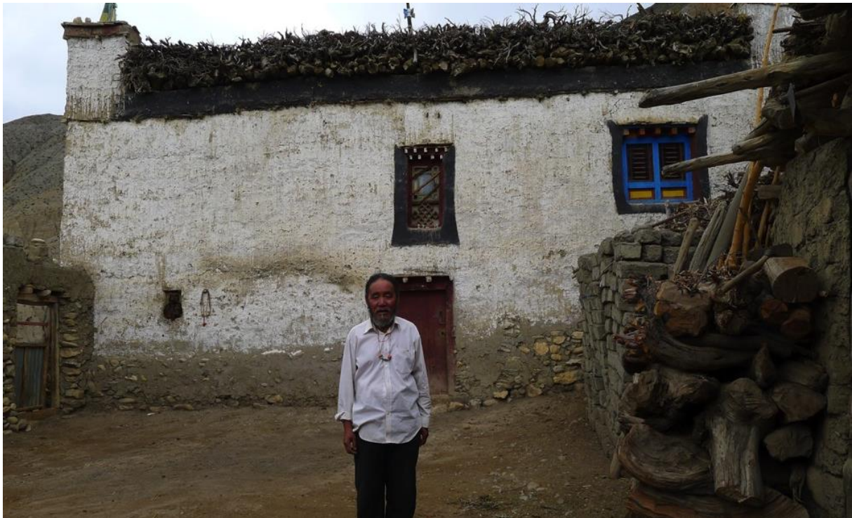
Figure 3.8: Outside view of a house in Dheye. The lower parts of the walls are made of stones whereas the upper parts are made of handmade earthen blocks, some of which are piled up on the right side of the house owner (photo: 06/07/2012, Daniel Pittet).
