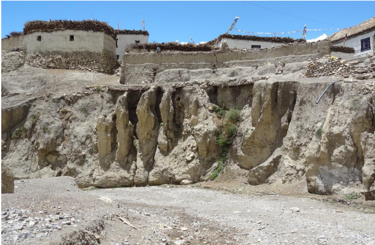
Figure 3.18: Gorge cliff within Yara exposing loose conglomerate and weathered chaotic rock mass. The gorge cuts through the village separating it into two parts. As can be seen, the bottom of the gorge accommodates the track to Ghara (photo: 04/07/2012, Daniel Bernet).
