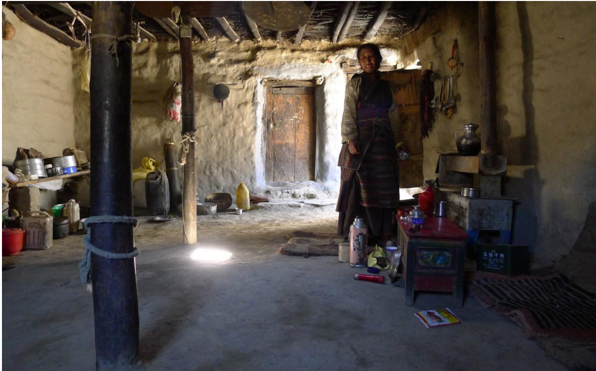
Figure 3.9: Inside view of a house in Samzong with earthen walls, wooden poles and wooden slab (photo 28/06/2012, Daniel Pittet).
