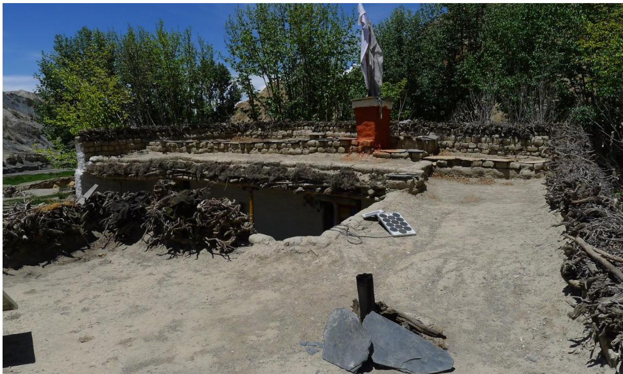
Figure 3.10: Roof top with soil/ash surfacing, wood disposal for drying, solar modules for lighting system, shrine (in red) and pipe for fire smoke evacuation in Samzong. The places corresponding to inside partition walls are covered by flat stones for a better protection against rainwater penetration (photo 28/06/2012, Daniel Pittet).
