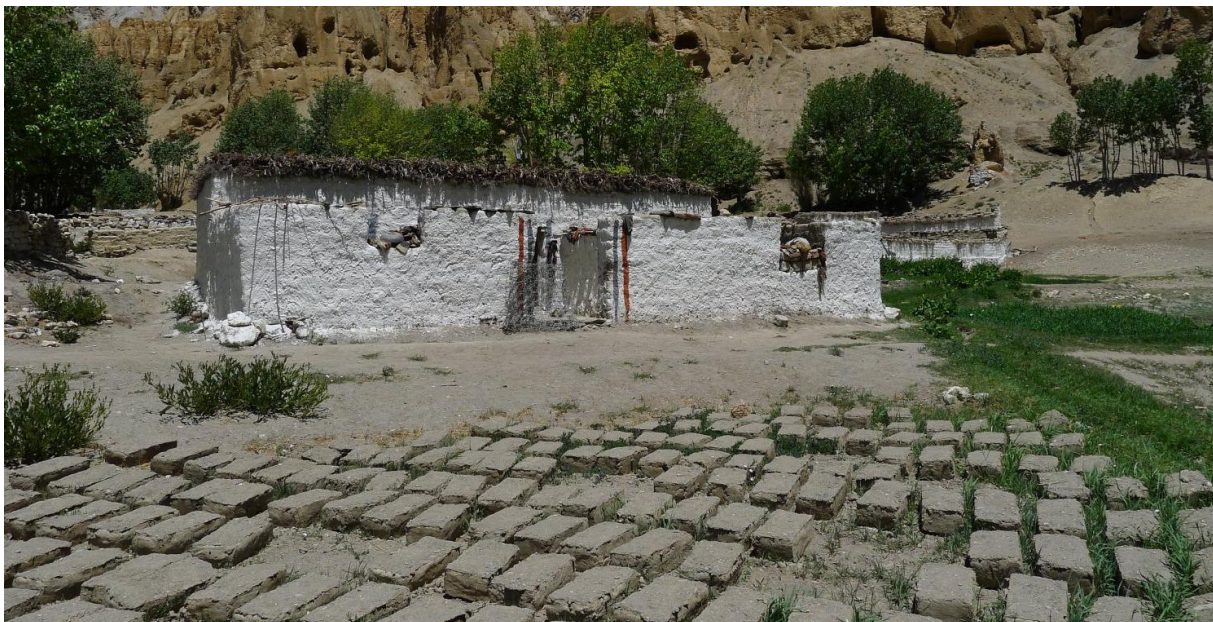
Figure 3.8: Hand-made crude soil blocs for wall construction in Samzong (photo: 29/06/2012, Daniel Pittet)
