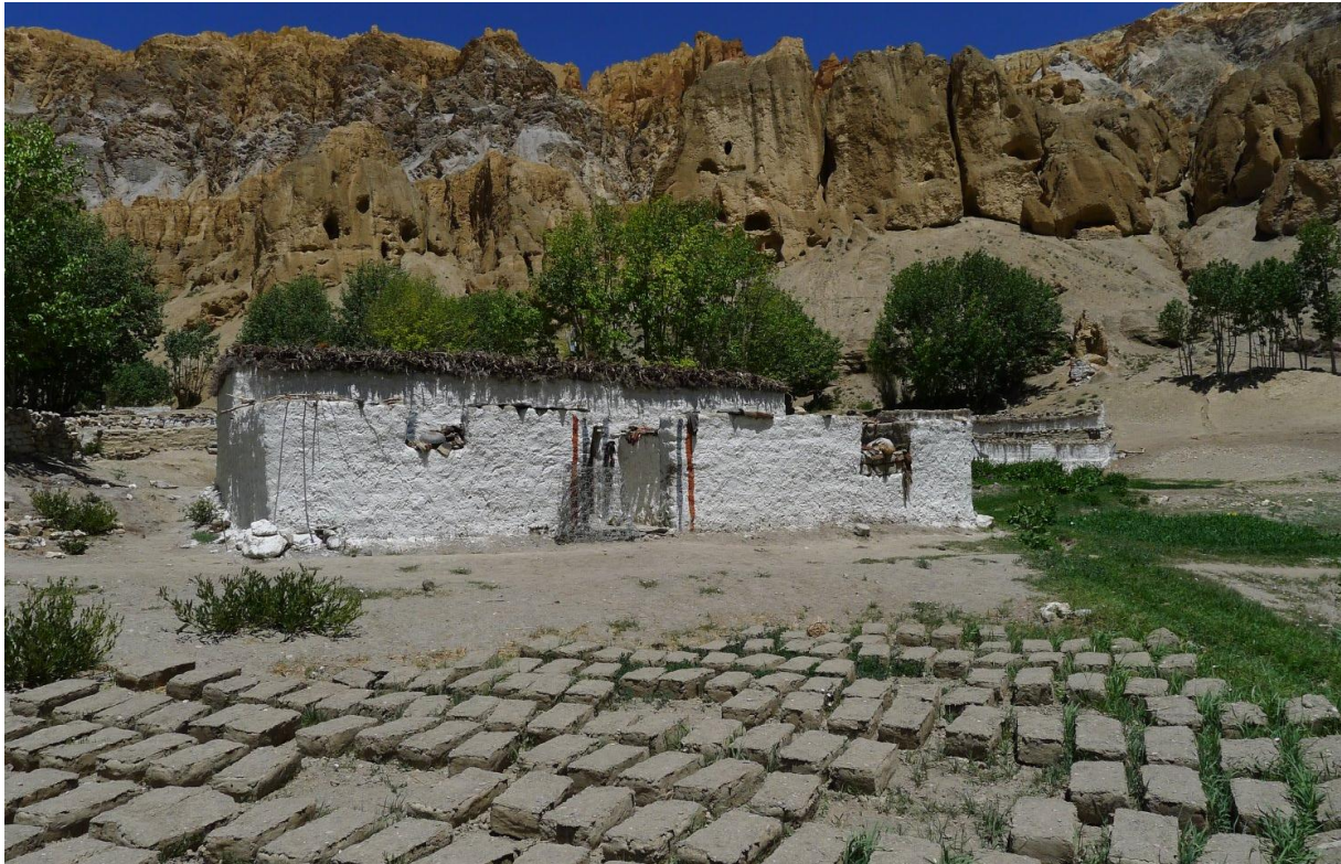
Figure 3.2: Hand-made crude soil blocs for wall construction in Samzong (photo: 29/06/2012, Daniel Pittet)
